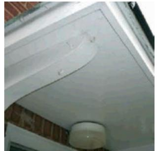
*Confirmed chrysotile (white) asbestos in ground floor external canopy soffit – manage only.*
