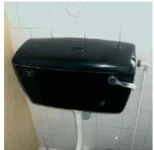
*Confirmed amosite (brown) asbestos in bathroom toilet cistern – manage only.*
