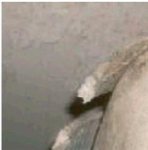
*Confirmed chrysotile (white) asbestos in asbestos cement water tank within 1st floor bedroom cupboard – manage only.*
