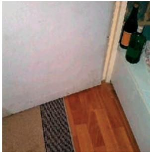
*Confirmed amosite (brown) asbestos to lining to boiler cupboard door – encapsulate, label and manage.*
