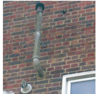
*Confirmed amosite (brown) asbestos to flue – encapsulate, label and manage.*
