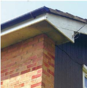
*Suspected asbestos cement boarding to first floor eaves soffit (guttering level) – manage only.*
