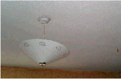
*Confirmed chrysotile (white) asbestos in textured ceiling coating – manage only.*
