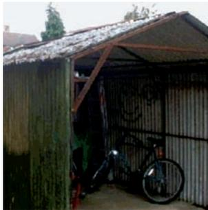
*Confirmed chrysotile (white) asbestos to garage walls and roof – manage only.*
