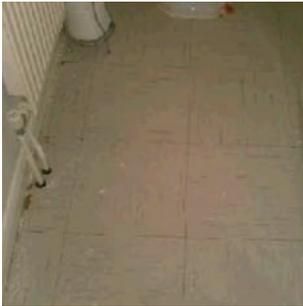
*Suspected asbestos in floor tiling in toilet – manage only.*
