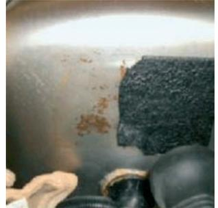
*Confirmed chrysotile (white) asbestos in ground floor kitchen bitumen pad beneath sink drainer – manage only.*
