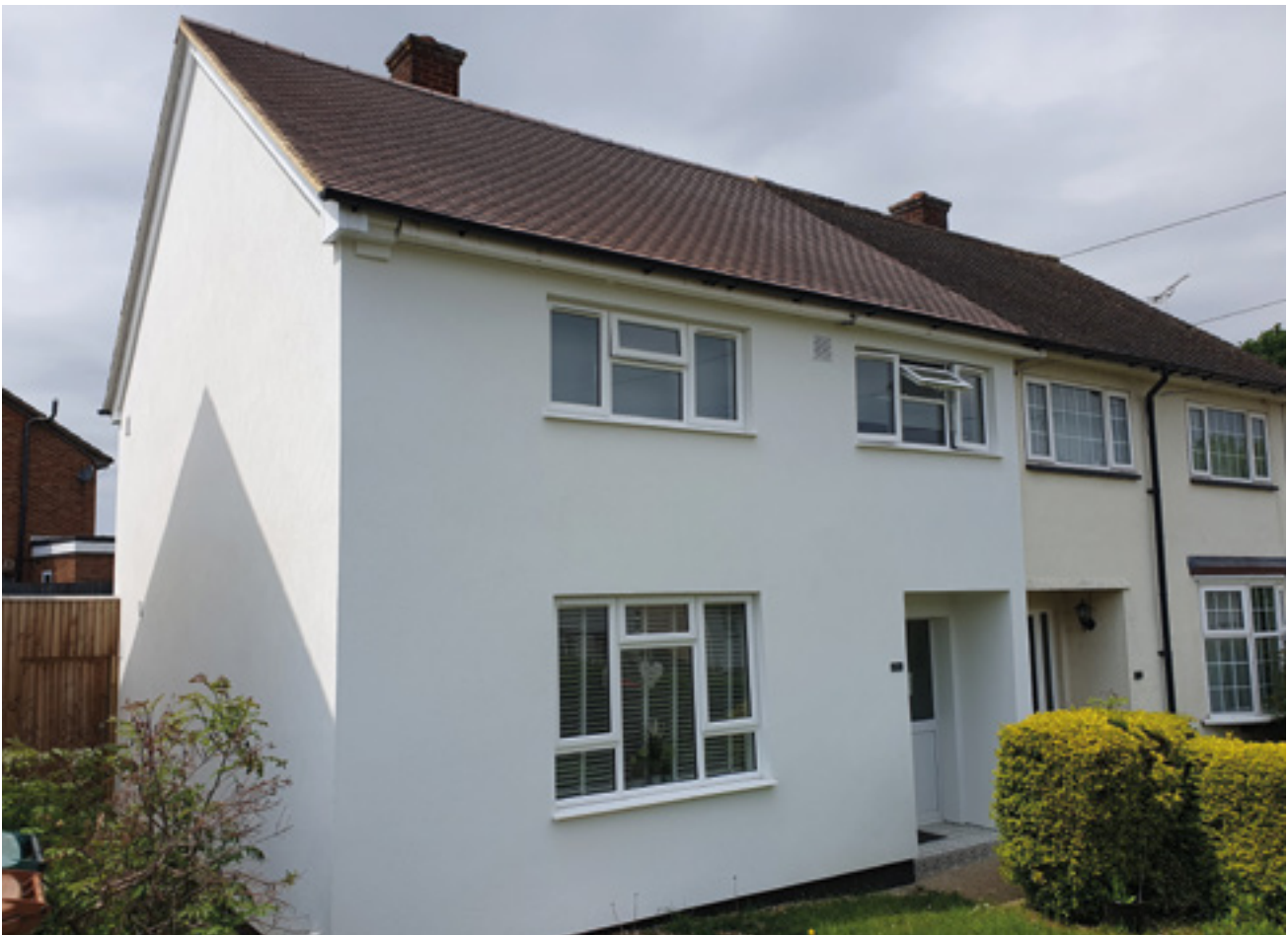
External wall insulation added to homes in South Oxhey with grant from Social Housing Decarbonisation Fund
